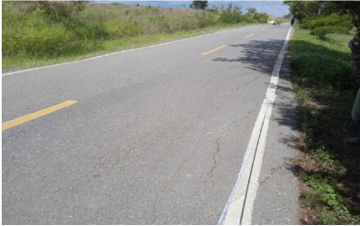
Gambar 7. Retak Halus (tracking).
