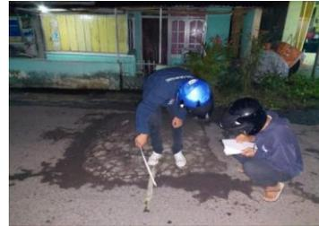
Gambar 4.6 Patching & Util. Cut Patching
