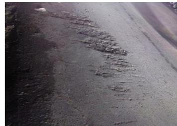
Gambar 4.7 Slippage Cracking
