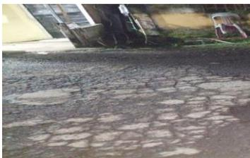
Gambar 4.4 Block Cracking
